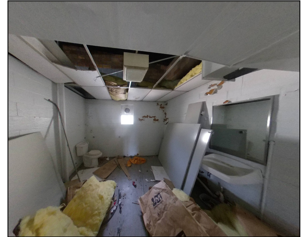
Fig. (012). Removal of plumbing fixtures in second level restrooms.
