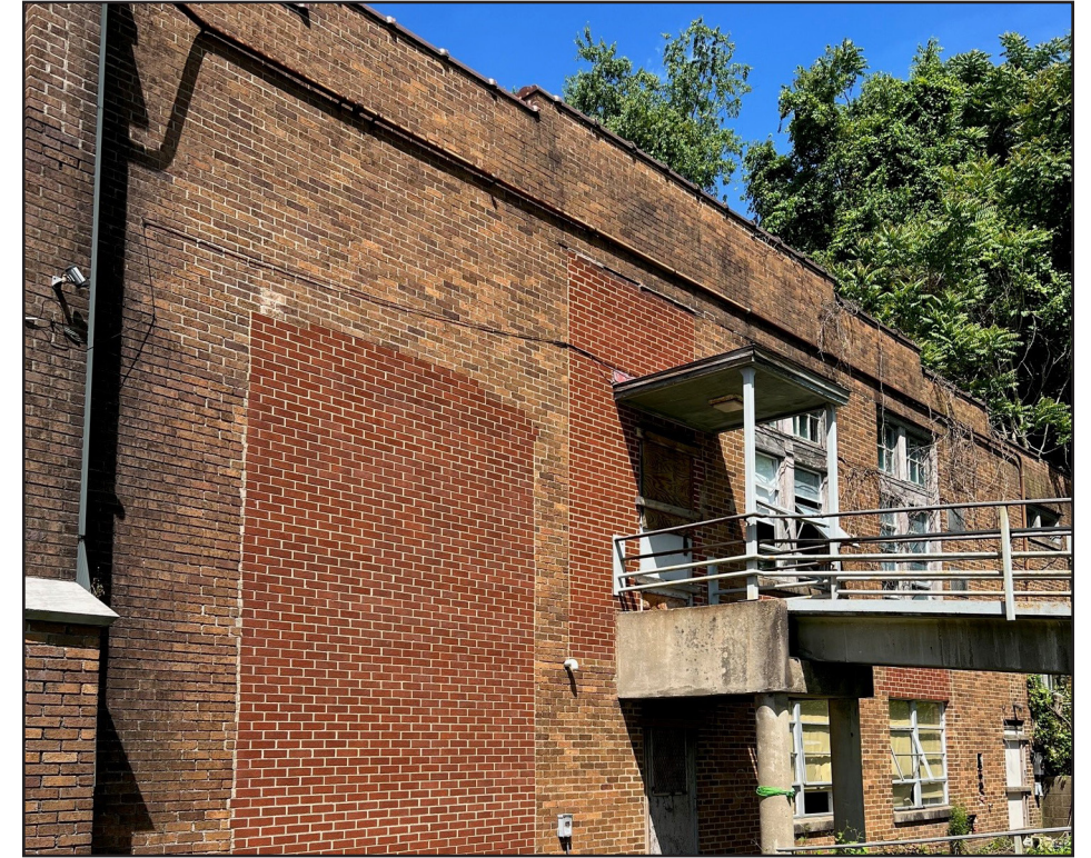
Fig. (017). The ramp landing on the south side of the building.
